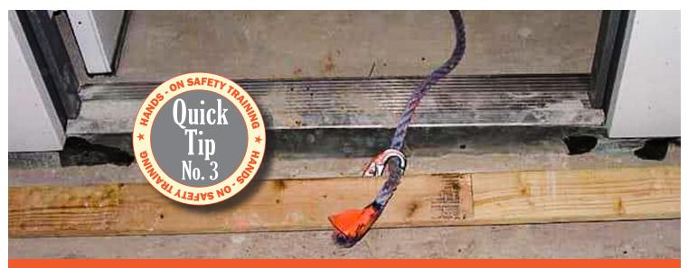
Your employees need to work on an unfinished balcony without guardrails, the interior of the unit has drywall installed and no place to tie-off. They had seen someone else using a door jamb anchor and they thought they could build their own.
